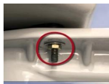
tank base bolts
