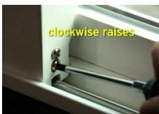
Adjust the clearance on a horizontal sliding window that is dragging by first taking off the weight by lifting the bottom of the window slightly and inserting a screwdriver into the access hole to adjust the rollers to the proper height. The lock strike may need to be adjusted as well after adjusting the rollers by loosening the strike screws and adjusting the height of the strike (up or down).
