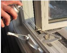
Lubricate window moving parts with a lithium multipurpose lubricant once or twice a year. Tighten and secure any screws.
