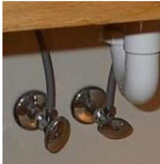
Once a year, fully operate the valves to the closed and opened position once or twice. When you are done, fully open it once more before closing it down a ¼ turn. Moving these valves sometimes releases loose sand or minerals into the water line to a faucet, so remove and clean a faucet aerator as well.
