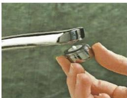
**Reinstall the aerator on the faucet.** Screw the aerator in by hand in a **counterclockwise** direction. Use the pliers to tighten securely if it leaks. There is no need to over tighten. Snug is good!
