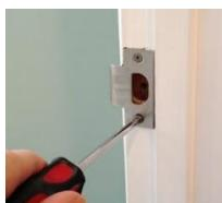
If a door does not close tightly usually the door stop or strike plate (metal plate where the door latch goes into the door frame) is loose. Securing the door stop or tightening the strike plate should help. If the door is not latching properly. The strike plate may need to be adjusted.
