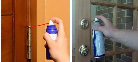
Annually lubricate hinges, lock sets, latches and dead bolts with white lithium spray grease and tighten screws. As an alternative graphite can be used to lubricate the lock set, latch and dead bolt. Rubbing a pencil on the key and inserting it into the lock then turning it a couple of times. Rub a pencil on the dead bolt or latch as well. If a hinge loosens between scheduled maintenance it is useful to tighten all the door screws and hardware as well.
