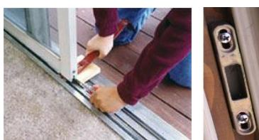
Adjust the clearance on a sliding glass door that is dragging by taking off the weight with a shim and inserting a screwdriver into the access hole to adjust rollers to the proper height (clockwise raises). Sliding screen doors may have adjusting screws on all four corners. The lock strike may need to be adjusted after adjusting the rollers. If the door will not latch loosen the strike screws and adjust the height of the strike (up or down).
