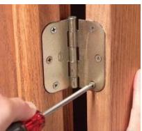
If a door rubs against the floor covering and/or is sagging try tightening the hinge screws. If this does not help replace the center screw in the upper hinge with a longer 2 ½ inch screw.
